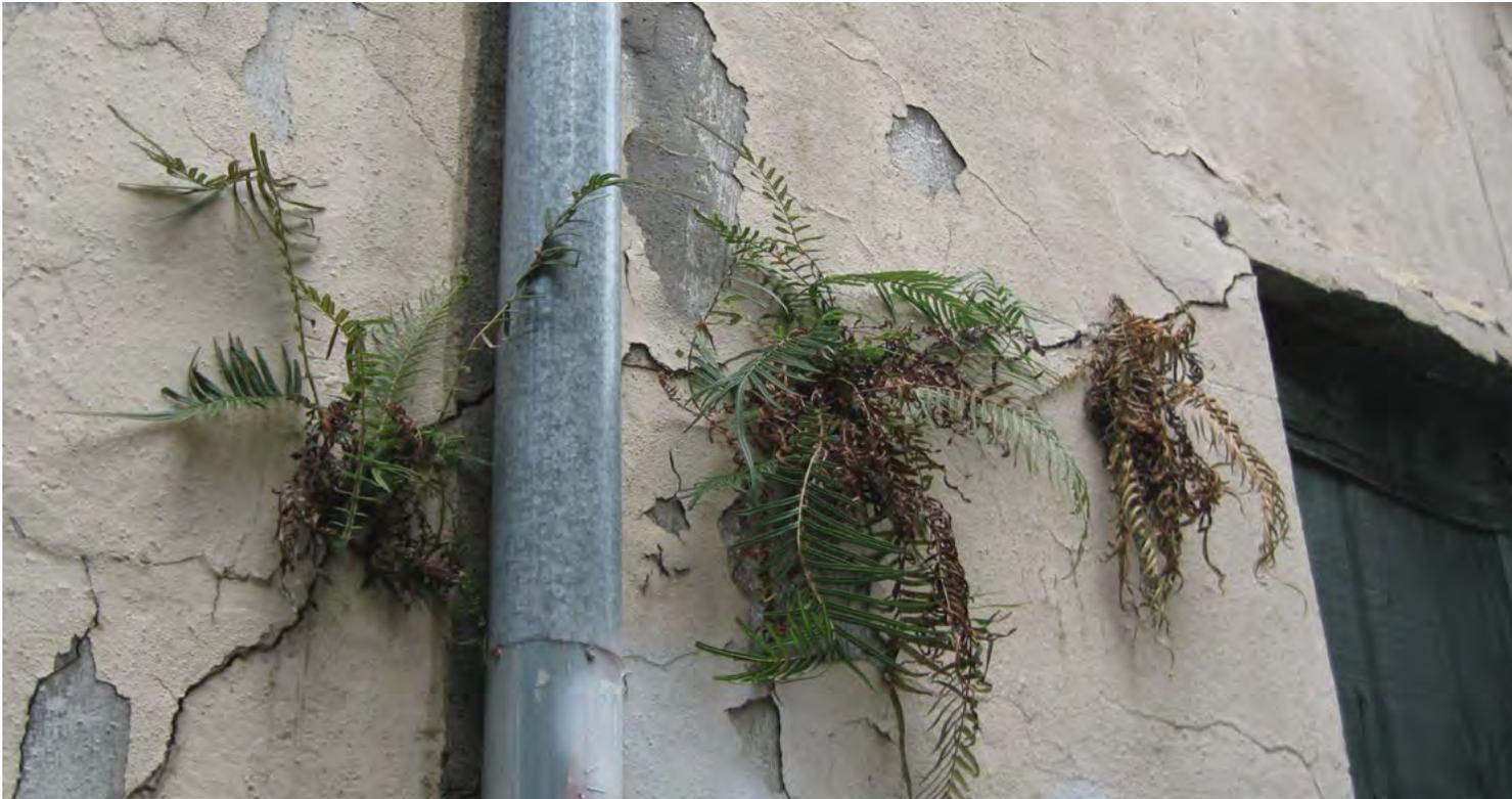
[3] **Not Recommended:** Cracks in the stucco have not been repaired, thereby allowing ferns to grow in the moist substrate which will cause further damage to the masonry.
