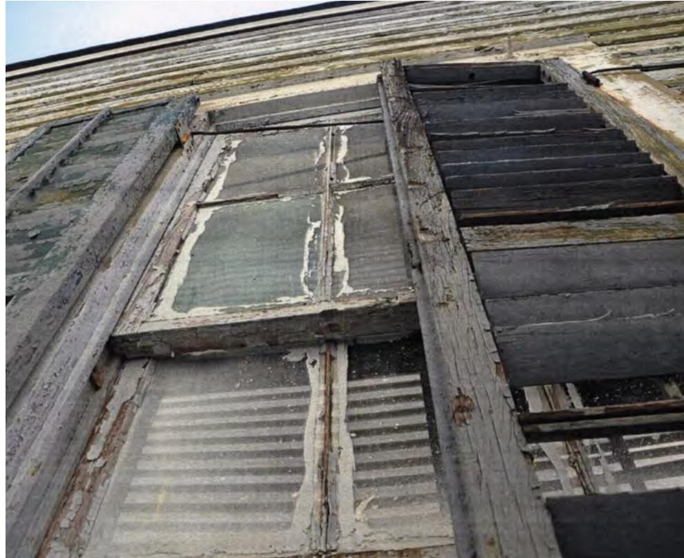
[11] Old and brittle glazing putty should be removed carefully before reputtying to keep window glazing weathertight.
