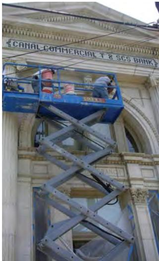
[1] An alkaline-based product is appropriate to use to clean historic marble because it will not damage the marble, which is acid sensitive.
